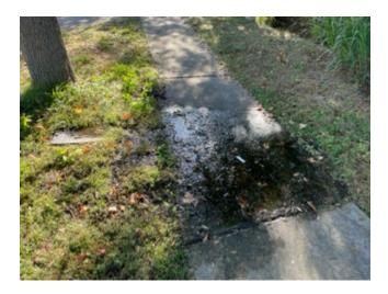
There appears to be an irrigation leak at the southwest corner of Deer Chase Dr, it will be inspected by the irrigation technician.
