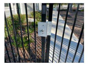
The magnetic lock on the gate appears to have broken off – Yellowstone screwed it back on temporarily at their last visit but it will need to be repaired properly.
